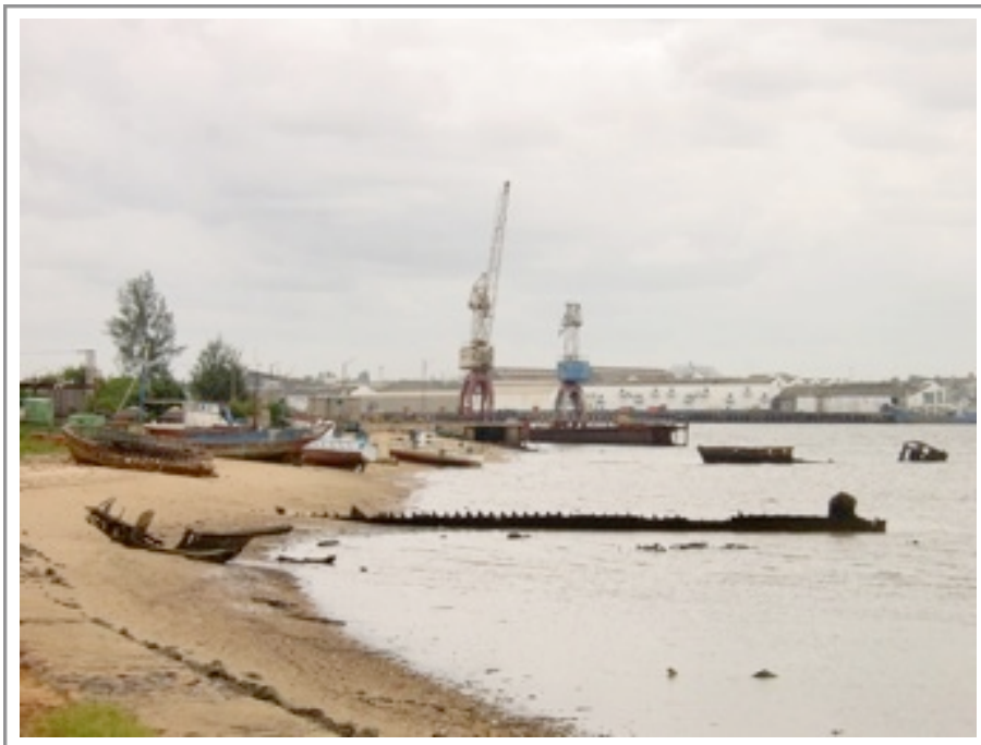
The dry dock in KaTembe with its two cranes
